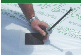
Install Nail Stakes on an Angle
