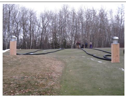
Installation of passive ventilation using whirlybird roof turbine to produce continual airflow
